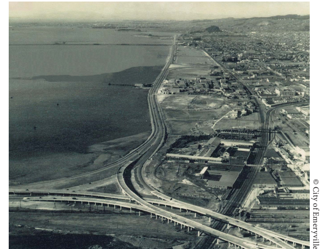
Developing on fill between the Eastshore Highway and the railroad, circa 1944.
