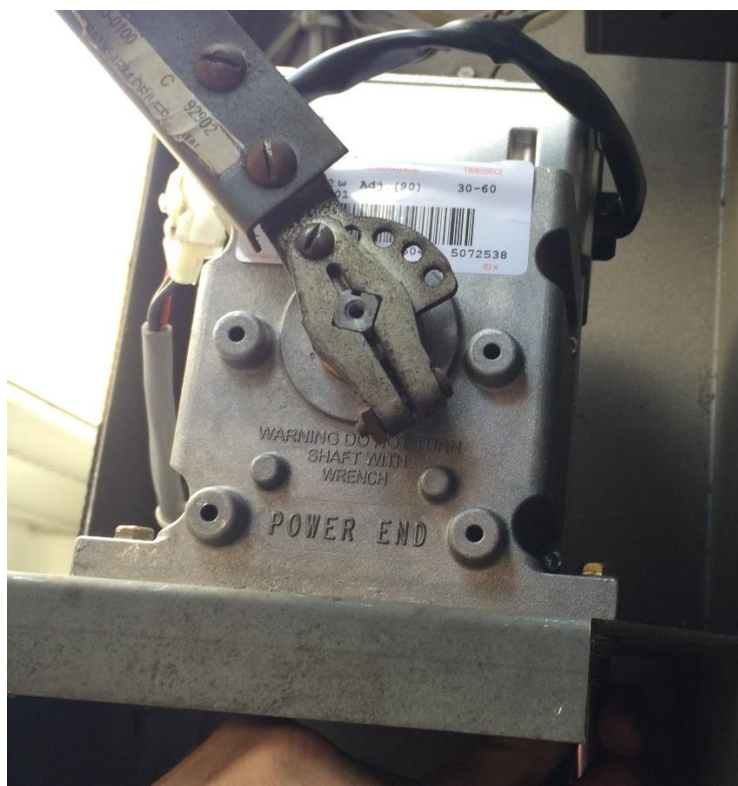
Figure 3.4: New Actuator Installed
