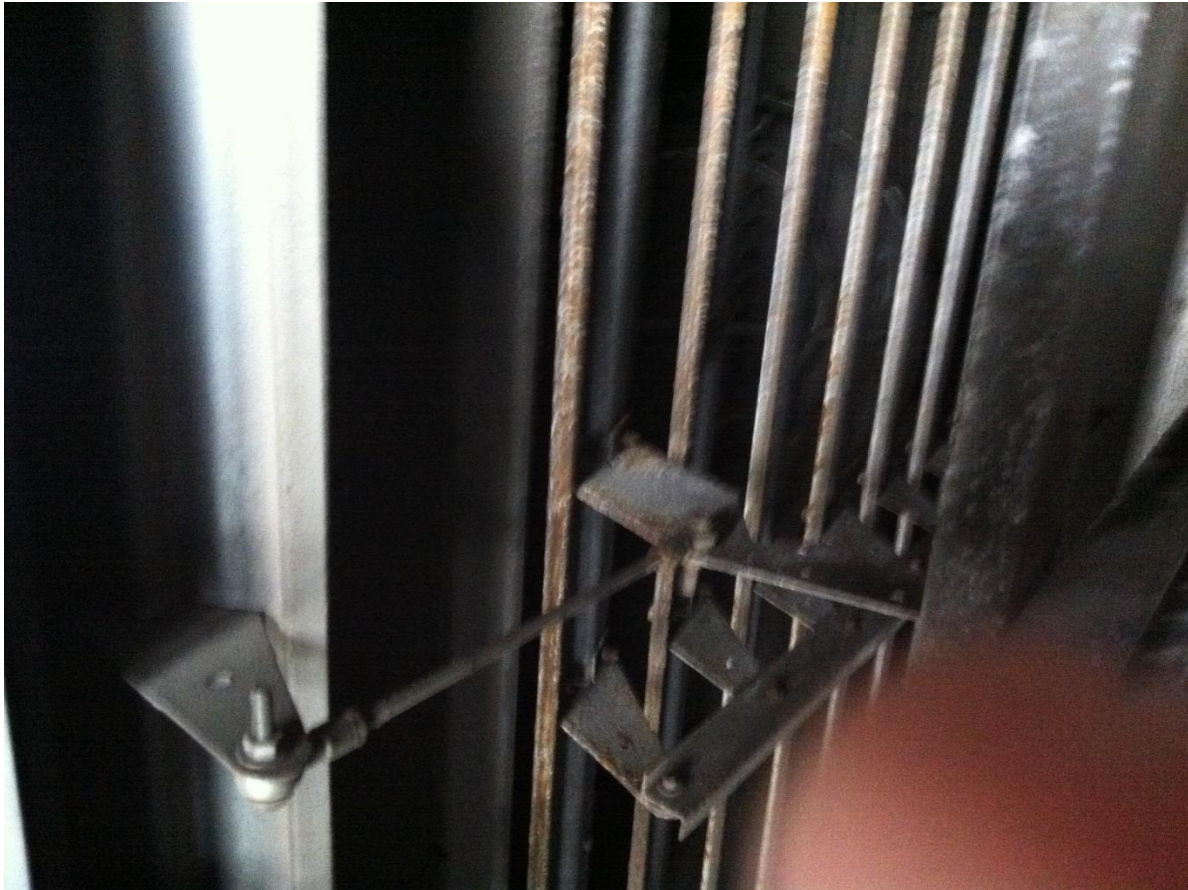
OA Damper set, Showing baseline linkage condition
