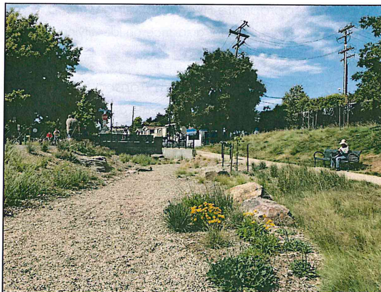
Figure C-6. Ohlone Greenway Natural Area and Rain Garden. This rain garden captures and treats runoff from an adjacent segment of Fairmont Boulevard. In this instance, the rain garden location provided an opportunity to convey and treat stormwater outside the street right-of-way. Source: PlaceWorks
