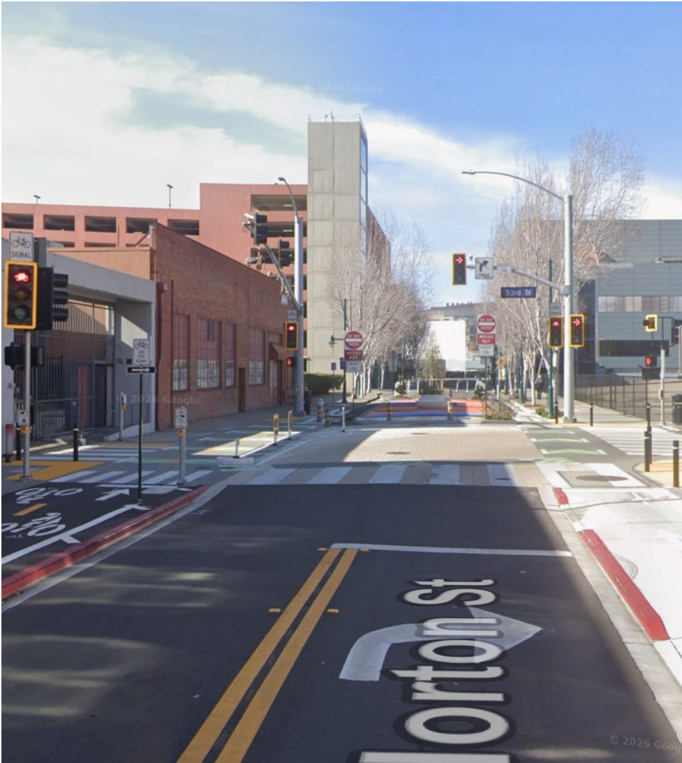
Horton Street and 53rd Street Traffic Diverter (looking north)
