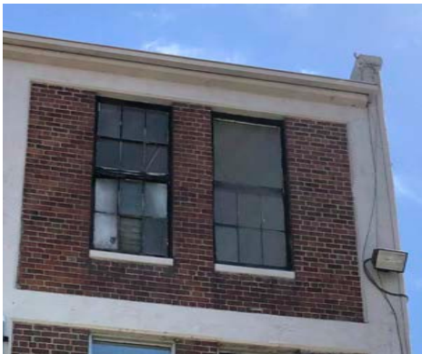
(E) single, double hung wood frame window
