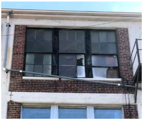
(E) double hung wood frame window
