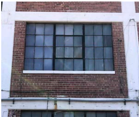
(E) typical industrial steel sash window
