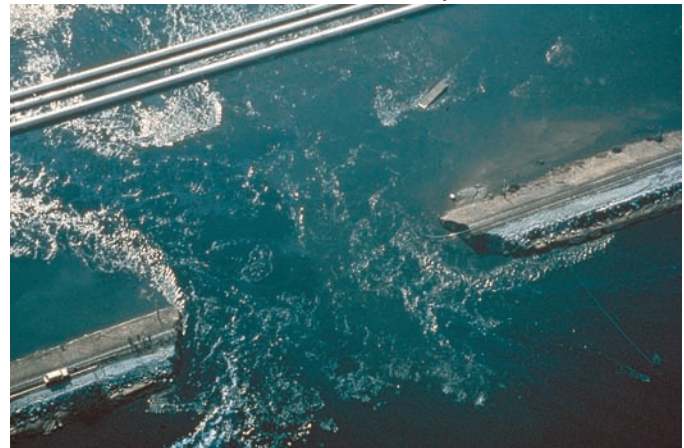
FIGURE 2-6 LEVEE FAILURE ON THE LOWER JONES TRACT IN 1980
