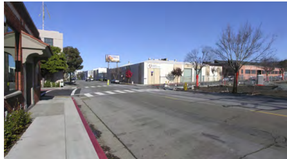
Utility Wires Undergrounded
