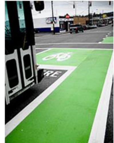
A ‘bike box’ provides colored pavement and an advanced stop line for automobiles. The bike box reduces conflicts at intersections by providing space for bicyclists to visibly position themselves ahead of motor vehicle traffic for either through or turning movements. Note also the pigmented/dotted bike lane treatment carried through the intersection.
