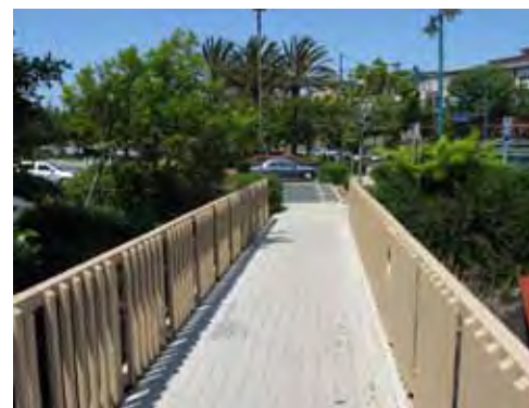
Bridge over Temescal Creek at Site H
