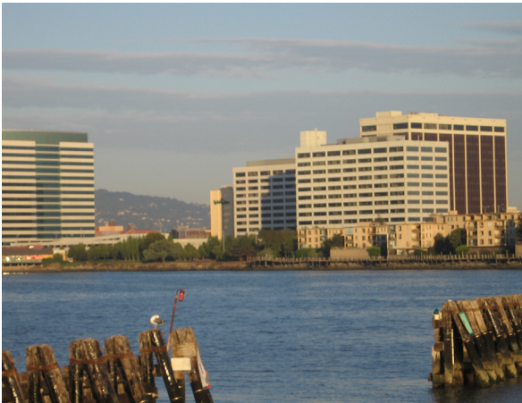
Artificial fill atop bay mud, along the shoreline of Emeryville may be susceptible to violent earthquake shaking.
