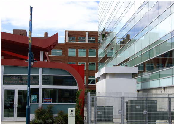
Construction activity (top) is restricted to certain hours of the day, but still causes short-term temporary noise impacts. Mechanical equipment that is not appropriately shielded or integrated into building design may lead to unnecessary noise exposure (bottom).
