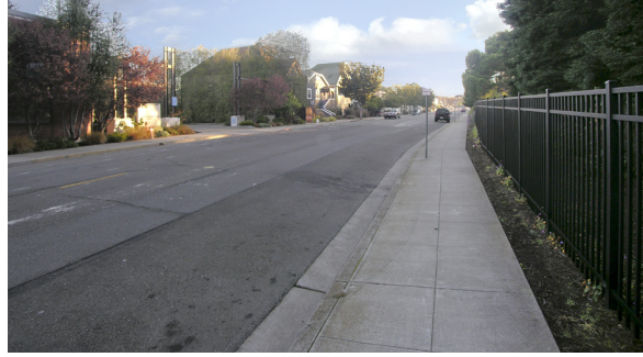
Utility Wires Underground
