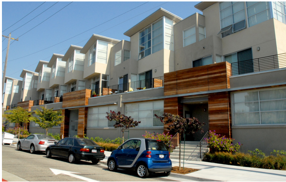
Taller slender buildings can allow opportunities for public spaces, mid-block connections, and more sunlight (top, San Francisco). Buildings with larger footprints may prevent them (middle). Buildings should step back on upper floors to create public or private open spaces and allow light onto the sidewalk (bottom).
