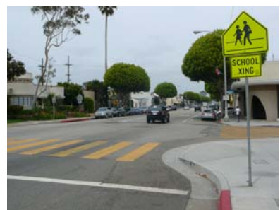
Curb bulb-outs improve visibility of pedestrians at the intersection.
