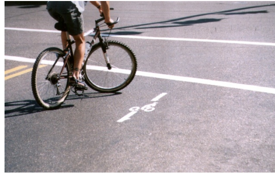
Type "C" loop detector in use in California.
