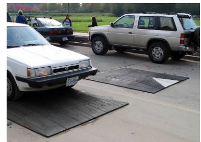
Speed lumps or cushions are divided to allow emergency vehicles to pass unaffected.
