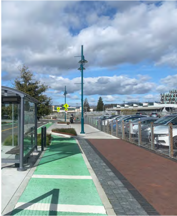
A raised bicycle lane next to the sidewalk on Shellmound St allows for people walking and rolling to comfortably share the same space.
