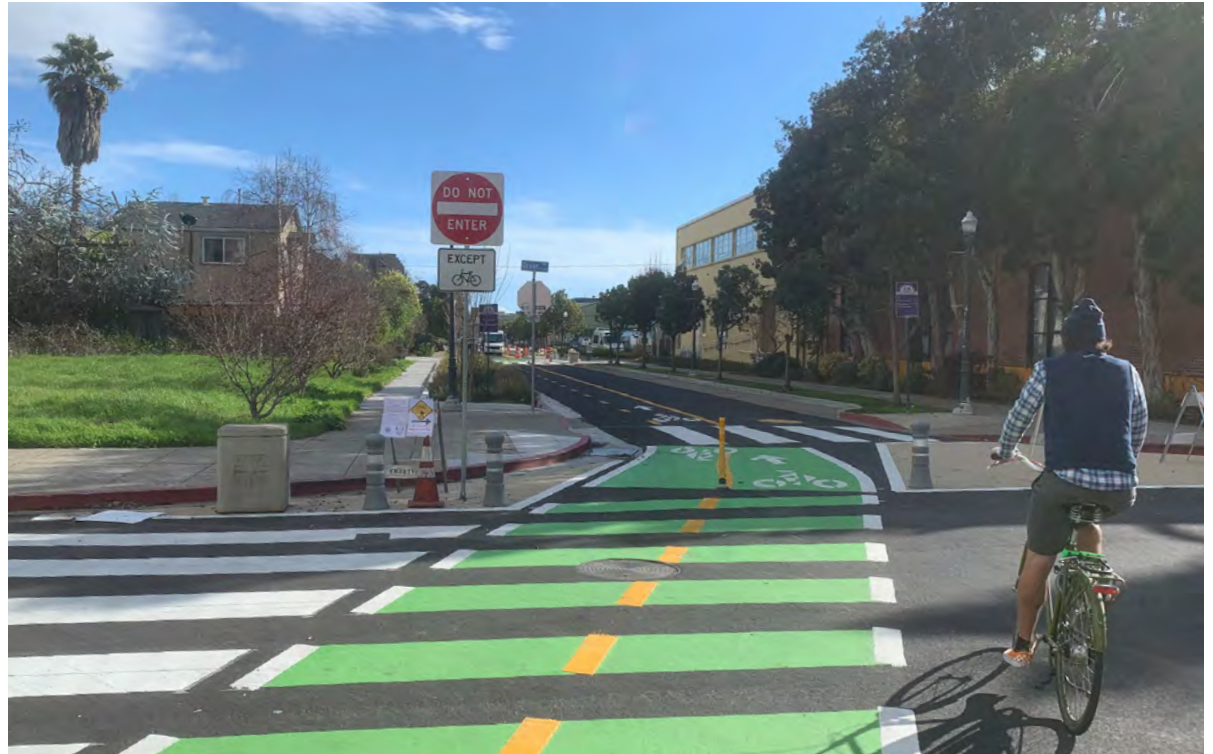
The Doyle Slow Street restricts access to cars in some locations, creating an on-road biking and rolling facility that is comfortable for all ages and abilities.
