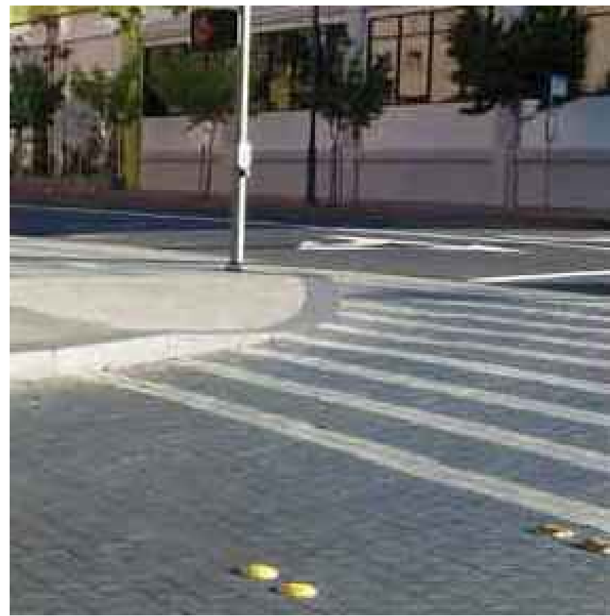
DARK GREY CONCRETE PAVERS WITH CONTINENTAL BANDING IN ELASTOMERIC WHITE PAINT, FLASHING LED SAFETY LIGHTS
