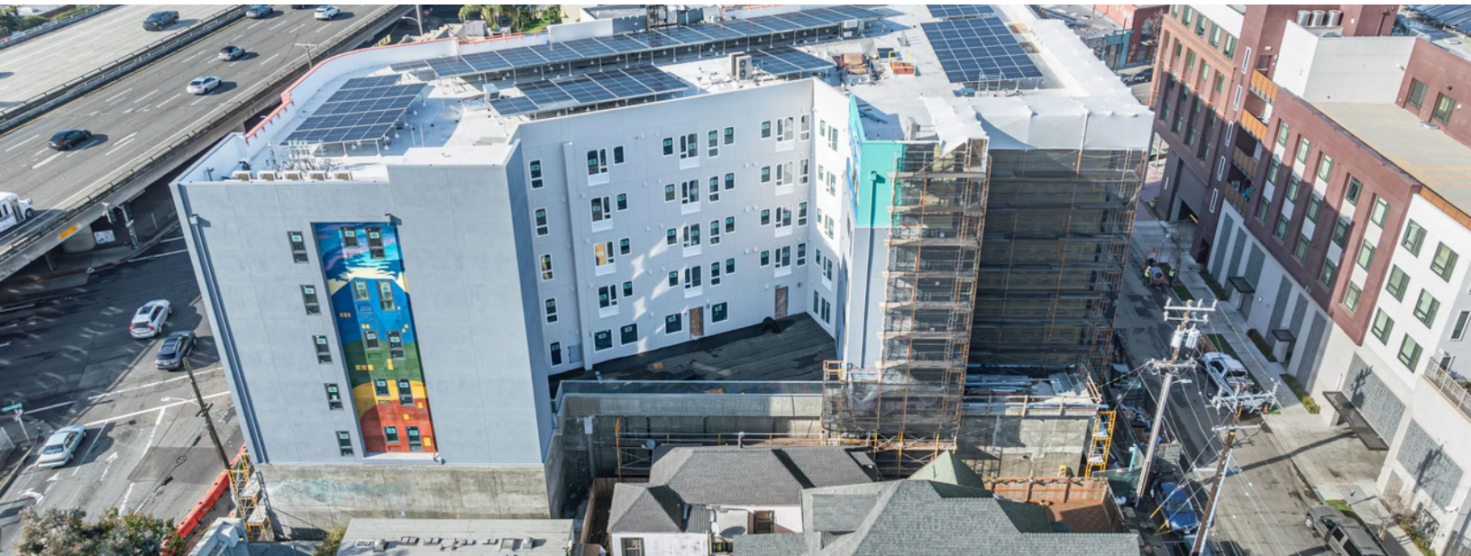
Nellie Hannon Gateway Apartments Under Construction
