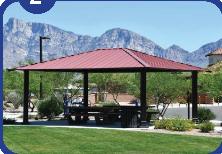
Metal Frame with Solid Ribbed Metal Roof
