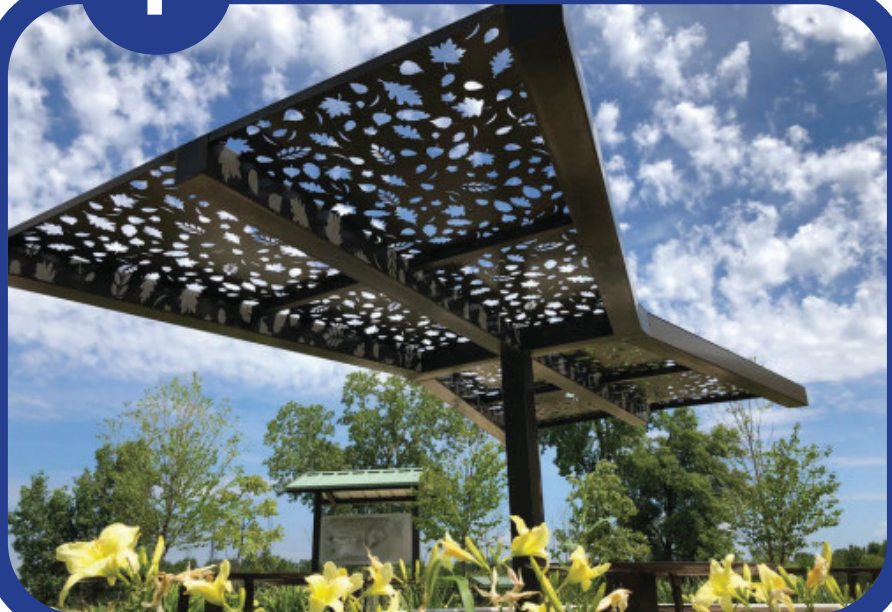
Metal Frame with Perforated Metal Roof
