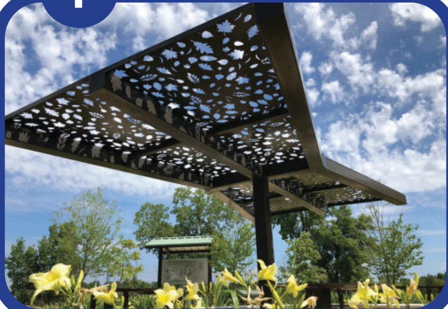
Metal Frame with Perforated Metal Roof
