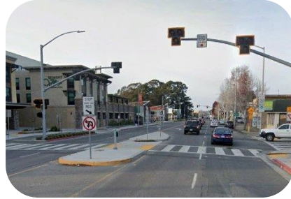
Signals/beacons & median refuges
