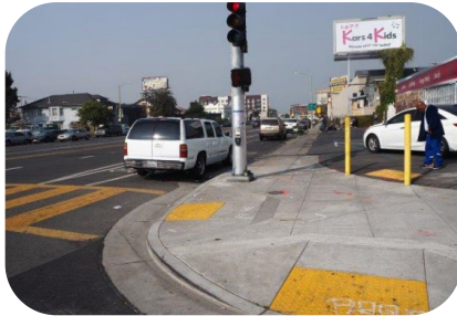
ADA ramp and signal upgrades
